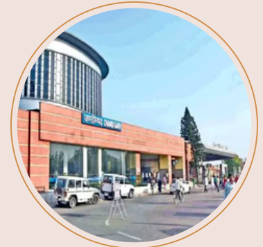
Chandigarh Railway Station
